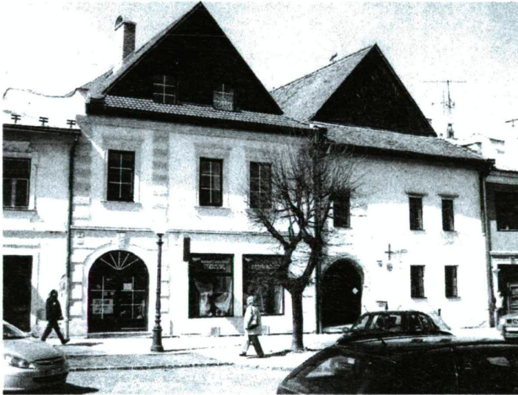
Fig. 3. An example of photographs taken in Kezmarok and listed in Fig.2 (KEZ 43) (Hric 2008)
